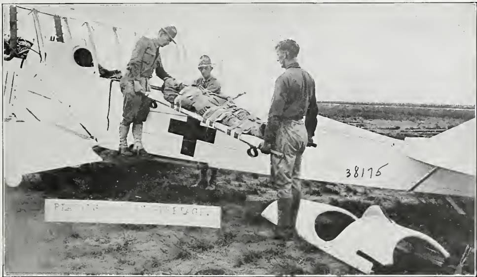
FIG. 146.—JN-4H airplane ambulance. Placing patient in fuselage, Ellington Field.
